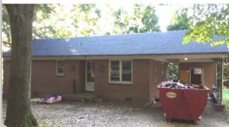
The renovation of the house on the new property is progressing. A new roof was installed last weekend! A big thanks to all who risked life and limb to remove the old shingles and install the beautiful new onyx black architectural 30 year shingles. The bathroom has been gutted and rotted wood repaired. The old carpeting was pulled out and sent to the dump. A new HVAC system will be installed in the coming weeks as well as a new hot water heater.
